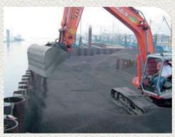
It has been effectively used to solve numerous geotechnical engineering problems and to convert unstable soft soil into usable land. Lightweight fill also provides permanent non-degradable insulation around pipe lines, and other thermally sensitive elements.
